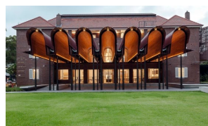
Heritage Buildings are celebrated with adequate curtilage and quality activation. Location: Joynton Ave Creative Precinct: Peter Stutchbury Architecture in association with Design 5 Architects
