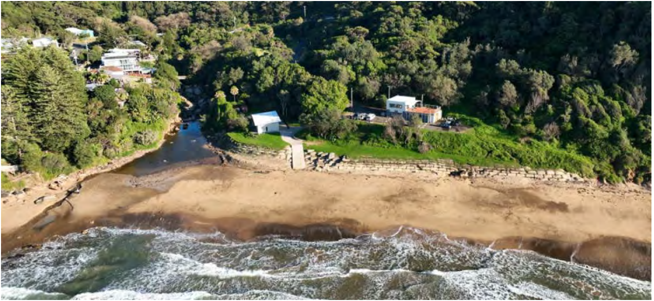
Figure 3.15 GSC seawall structure (image source: Salients, 2026)
