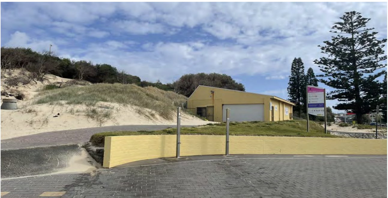
Figure 3.65 Wind-blown sand blocking a SLSC storage building at Port Kembla Beach
