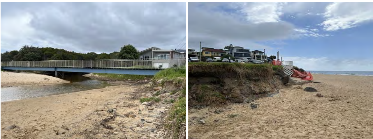
Figure 3.32 Entrance instability at Hewitts Creek impacting safe beach access. Image taken November 2025.
