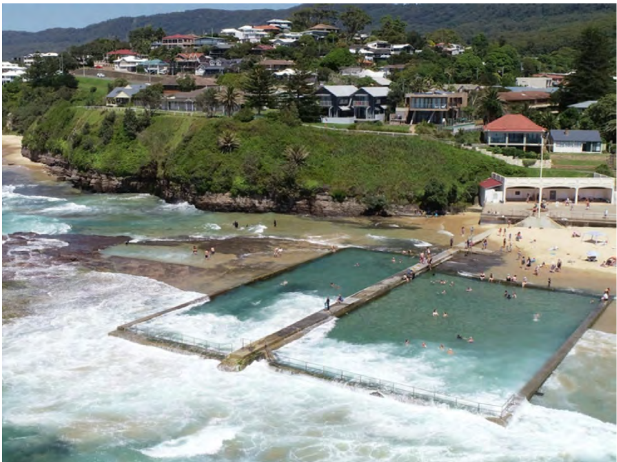
Figure 3.27 Wave overtopping of the Austinmer ocean pool (image source: WCC)
