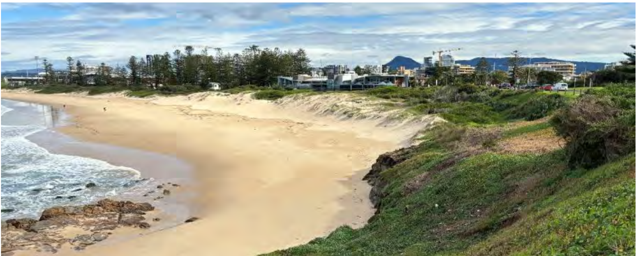
Figure 3.57 Wind-blown sand drift impacting dune vegetation at the northern end of City Beach (image source: Salients, 2026)
