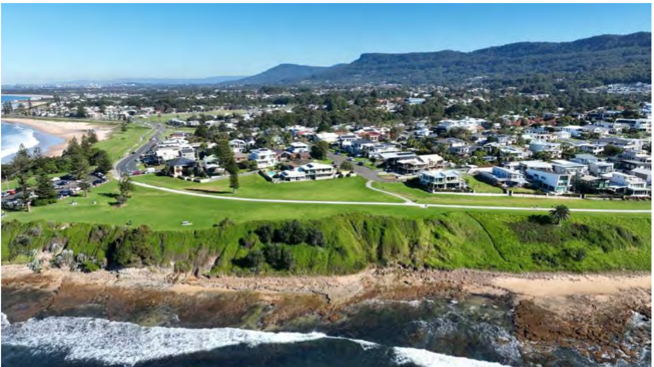
Figure 3.30 Southern end of McCauleys Beach (image source: Salients, 2026)
