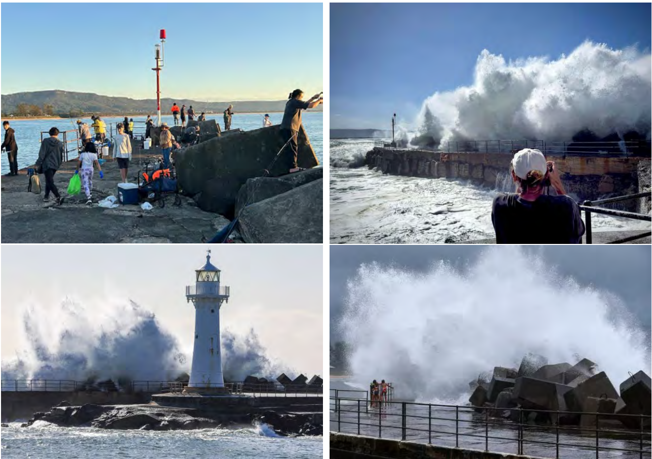
Figure 3.58 The Harbour breakwaters are popular recreational access spot, but are also subject to periodically dangerous wave overtopping (image sources: The Illawarra Flame)
