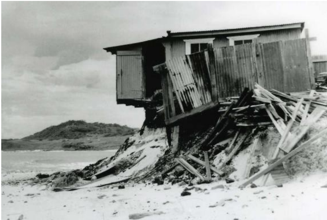
Figure 4 Erosion following Storms in the mid 1970's, Northern End of MM Beach 3
